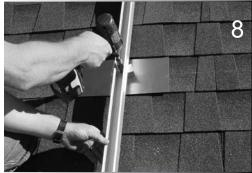
Using the Racking Hardware, secure the rack of your choice. Tighten to 16 foot pounds.
