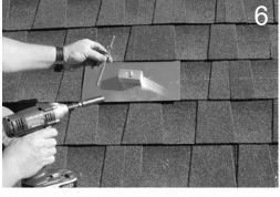
Slide Mount back into position. Prepare Hanger Bolt with 1 Hex Nut and 1 Sealing Washer, insert through Block into hole and drive Hanger until Block is tight.
