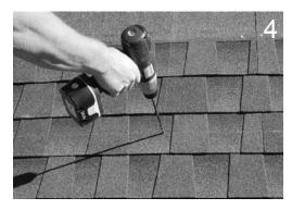
Using drill with 1/4" long bit, drill pilot hole into roof and rafter, taking care to drill square to the roof.
