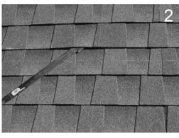
Lift Composition roof shingle with Roofers Bar, just above placement of Quick Mount.
