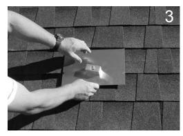
Slide Mount into desired position. Remove any nails that conflict with getting Mount flush with front edge of shingle course. Mark center for drilling.
