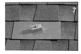
Insert EPDM Rubber Washer over Hanger Bolt into Block.
