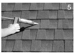
Clean off any saw dust, and fill hole with Seal-
